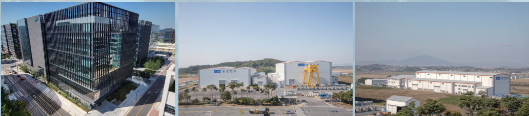
Magok Inno Center Hongseong Transformer Factory Hongseong Circuit Breaker Factory
